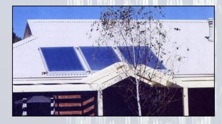
Designed to provide maximum solar contribution from Australian made & owned "Wise Living" flat plate solar thermal hot water collectors.
